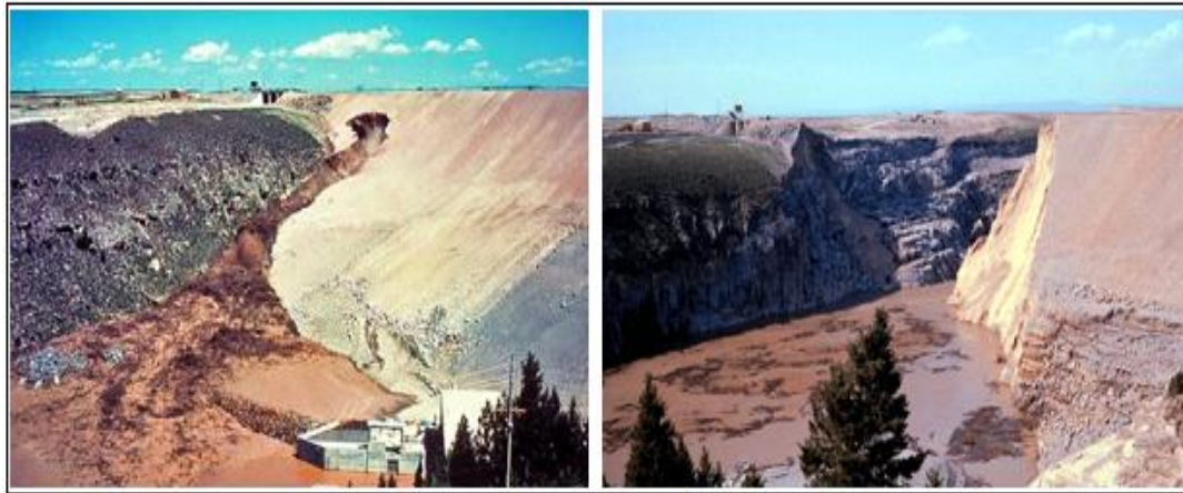
A. Beginning of Teton Dam breach
