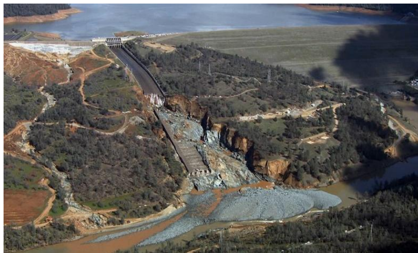
Figure (5): Oroville Dam spillway failures, February 2017
